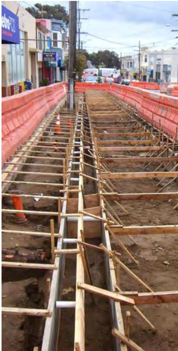
*Leland Avenue, San Francisco, under construction. Permeable pavement will be installed on the sidewalk and in the parking lane.*
