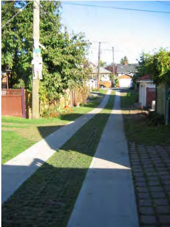
*“Country Lanes” in Vancouver, British Columbia enhance the alley’s aesthetic quality and reduce stormwater discharge to the City’s stormsewer system by allowing runoff to flow over vegetation and infiltrate into the ground.*
