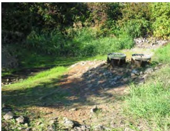
*An infiltration basin in Waterworks Gardens at the King County East Division Reclamation Plant, Renton, WA, is part of an environmental art park that treats stormwater. Runoff flows through stormwater treatment ponds, and the wetlands form an earth/water sculpture that funnels, captures and releases water.*
