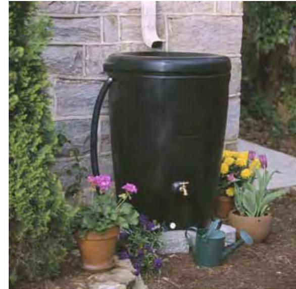
*A disconnected downspout and rain barrel.*
